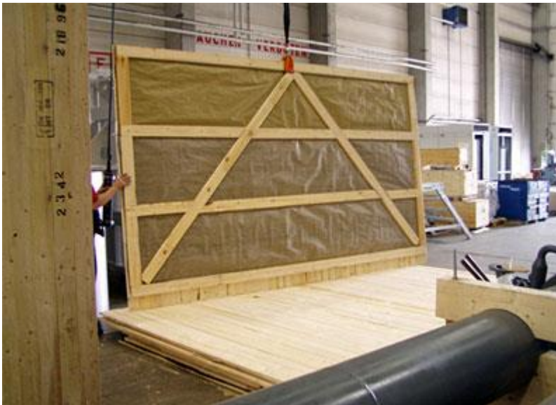
Figure 7: Side wall lined with a barrier layer
