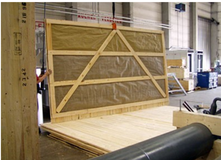
Figure 7: Side wall lined with a barrier layer
